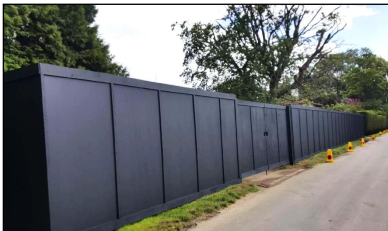
Figure 7.1 – Typical Site Hoarding Arrangement
