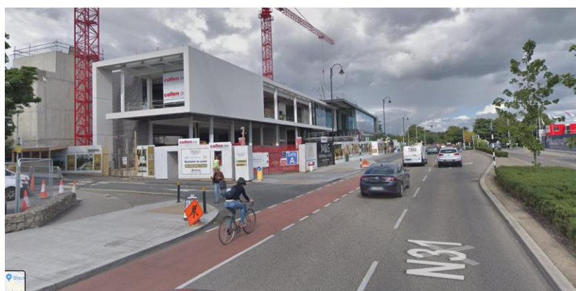
Photo 7.1 – Existing Site Access onto Frascati Road, looking north.
